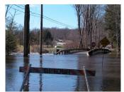
But while the waters from the Saugatuck River breached the bridge on Monday, the bridge maintained its structural integrity. "The new bridge was designed so water would flow over it when the river floods," Sgt. Brodacki said.
